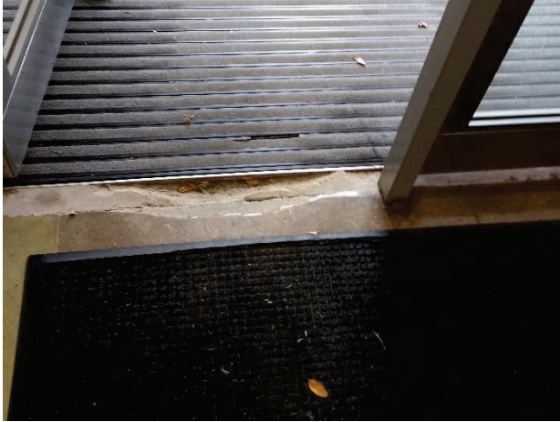
7. Threshold at entry is damaged. Walk off mat is worn.
