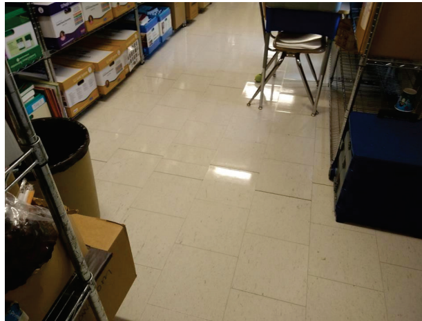
14. Vinyl floor tiles in Modular addition show signs which may indicate issues with subfloor.
