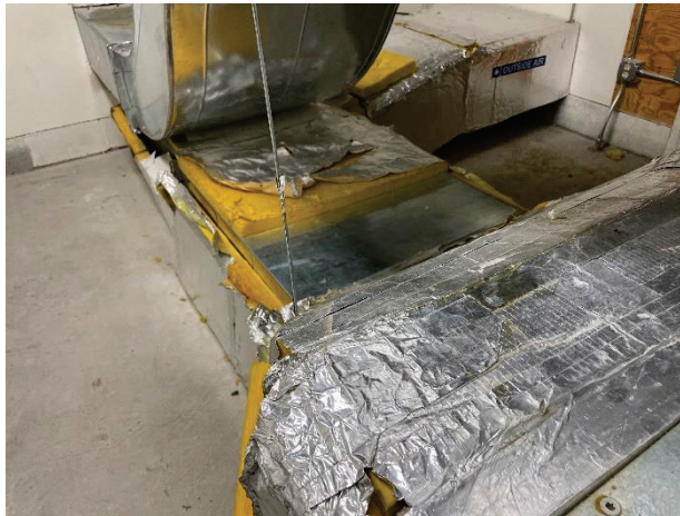
11. Some duct work has damaged or missing insulation.
