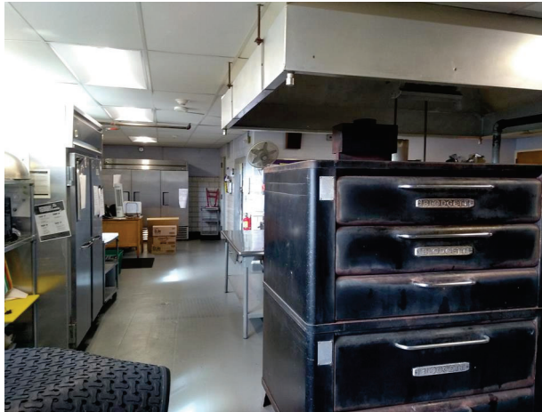
26. Kitchen equipment is very old and inefficient.
