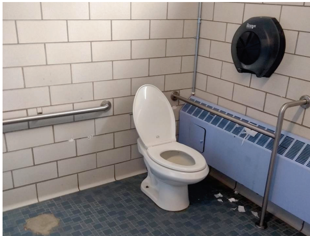
23. Grab bars/accessories are non-compliant and original tile floor is patched.
