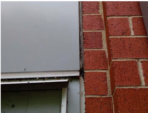
5. Sealant at metal panel is showing signs of deterioration.
